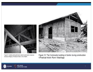
That is where you see in the next slide, you can see that here that the joining of the beams and the columns, how carefully they have them because that is where, it is going to tie the whole building and it is going to make sure that the whole structure acts in a better way in terms of the earthquake, when earthquake happens and because when the canes are woven in a fashion it will also not only the aesthetic character of it but it also gives a kind of structural stability.
